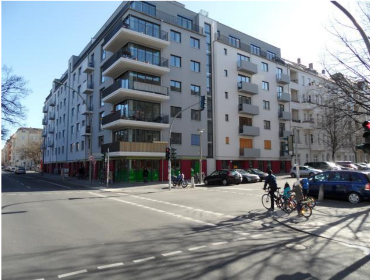
Passive house of 41 flats in Berlin, Arnimplatz
